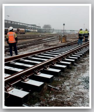
The hybrid polymer sleepers have been designed for longevity, not only to reduce the Total Cost of Ownership, but also to maintain continuous track stiffness when used for interspersing with timber sleepers. The KLP® Hybrid Polymer Sleepers are ideal for selective replacement of timber sleepers as well as for use in areas where timber or concrete sleepers are not the most beneficial choice for your track.
